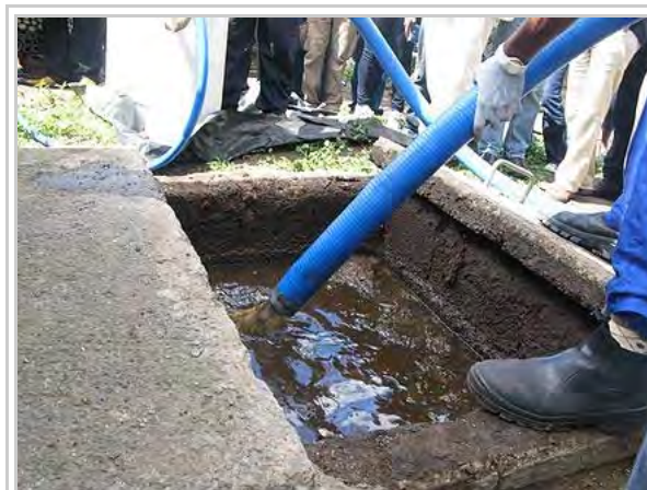
Demonstration of new equipment used for pumping fecal sludge from a pit latrine near Durban, South Africa
