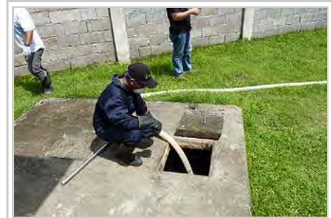
Desludging using proper personal protective equipment in Dumaguete, Philippines
