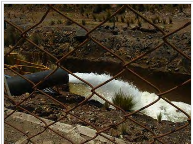
Industrial wastewater effluent with neutralized pH from tailing runoff. Taken in Peru.
