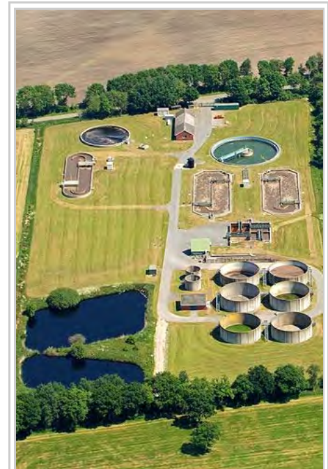
Wastewater treatment plant in Cuxhaven, Germany
