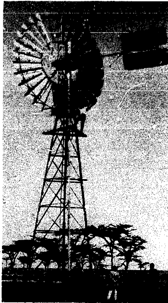
Fig. 1. Southern Cross windmill with a rotor diameter of 21 ft (6.4 m), installed more than 30 years ago.
