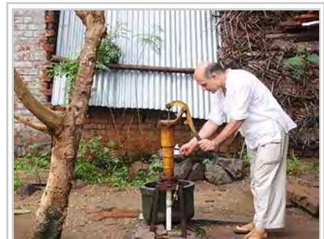
Hand pump to pump water from a well in a village near Chennai in India, where the well water might be polluted by nearby pit latrines
