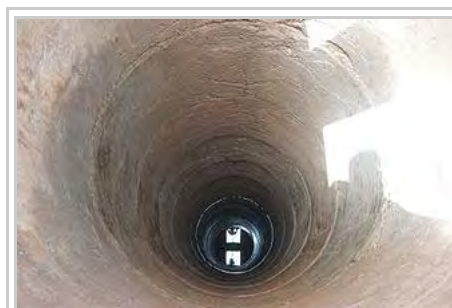
View into a hand-dug well cased with concrete rings; Ouelessebougou, Mali.
