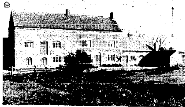
Fig 2.7 Holdenby, on a tributary of the North Water of the River Nene, and adjoining mill house. This is one of ironstone whereas most of the mills on the Nene West Water were of brick
