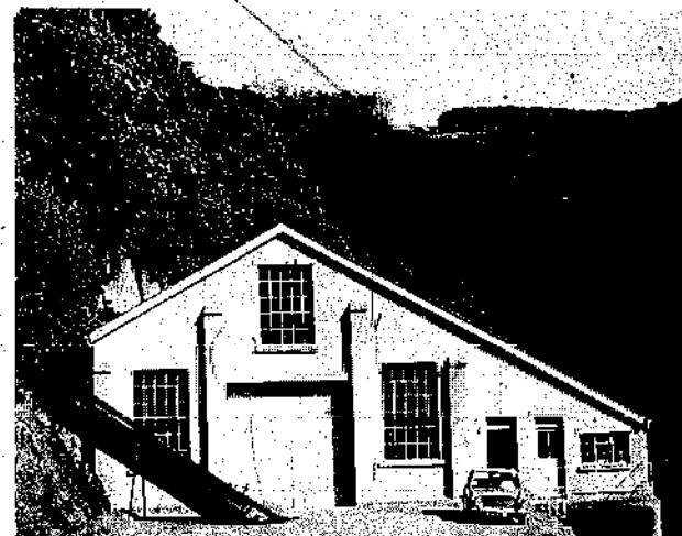
Fig 2.62 Morwellham generating station of the Central Electricity Generating Board. This is on the Devon side of the River Tamar and obtains approximately 20000 m 3 of water per hour from the disused Tavistock canal via the pipe which crosses in front of the bottom left of the building
