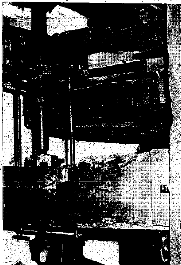
Fig 1.48 Iron stone nut and wooden great spur wheel at Billing Mill. The stone nut is held out of mesh by the jack ring supported by the two spindles passing through the wooden beam (or bridge tree) on either side of the bridging box carrying the footstep bearing for the stone spindle. When the jack ring is lowered by rotating the handle below the bridge tree, the stone nut descends to mate with the conical drive collar on the stone spindle and at the same time meshes with the cogs of the great spur wheel
