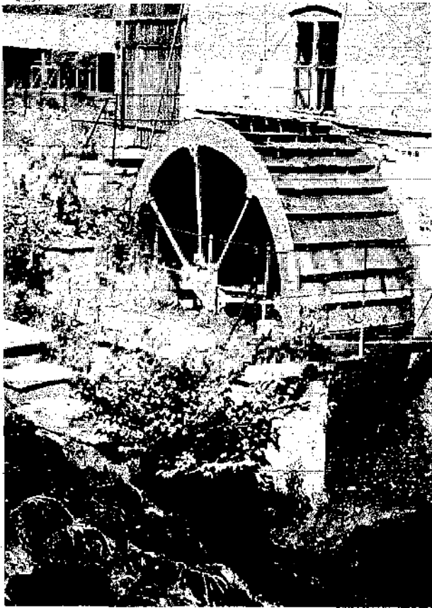
Fig 1.31. The breastshot wheel which used to drive the corn mill at the end of Arkell's Donnington Brewery, near Stow-on-the-Wold, Gloucestershire
