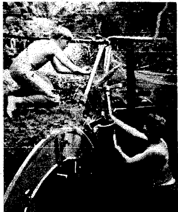
Fig 2.40 Boys from Grenville College, Bideford, clearing debris from the launder serving one of the waterwheels at the Finch Brothers 'Foundry', Sticklepath, Okehampton. These works have not been restored and the waterwheels work again under the auspices of a charitable trust
