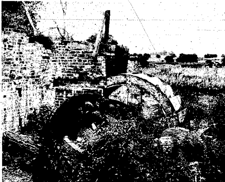
Fig 1.33 Overshot waterwheel in the ruined mill close to Clutchover, near Rugby, Warwickshire. Note the remains of the wooden launder and 'slut' for bringing water onto the top of the wheel
