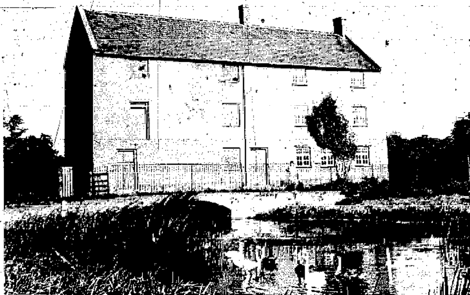
Fig 2.10 Upton Mill, on the River Nene west of Northampton, with the mill and millhouse under a continuous slate roof. The layout of windows and doors distinguishes the working part on the left from the domestic accommodation on the right
