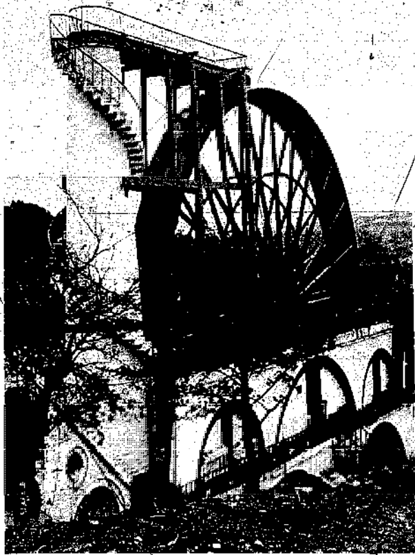
Fig 1.15 Pitch-back waterwheel at Laxey, Isle of Man. The water was supplied from a reservoir higher up the valley, the head of which is sufficient to raise the water up to the top of the circular tower and on to the launder serving the wheel. Note the stationary curved cover over the wheel near the tower, to prevent water being blown out of the buckets on the wheel. The crank, on the wheelshaft, is partly hidden by the tree in the foreground, but the connecting rod to the bell-crank lever and counterbalance weight is visible on the right of the masonry supporting the wheelshaft
