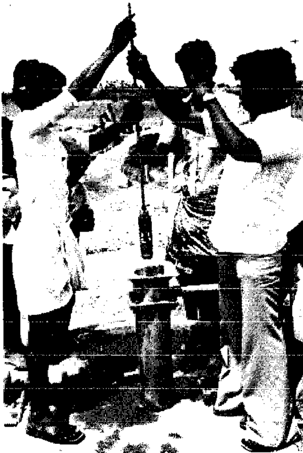
Village Level Operation and Maintenance — VLOM — of handpumps has a substantial effect on reducing recurrent costs. The alternative of centralized maintenance is the only option for motorized pumps.
