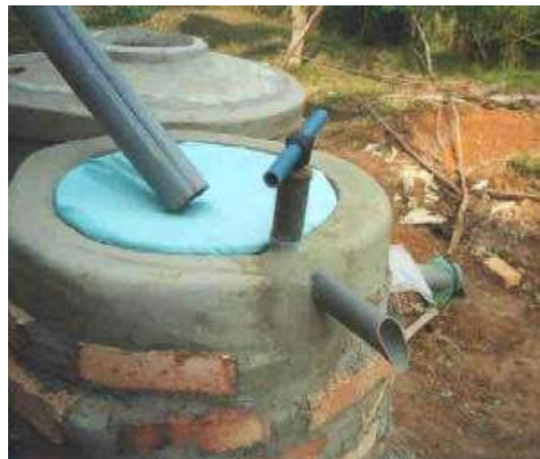
Figure 2 A Harold pump cemented into a plastic tube tank at Kyera Farm
