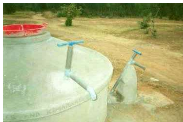
Figure 4 The DTU (left) and the Tamana handpumps fitted to a partially below ground tank
