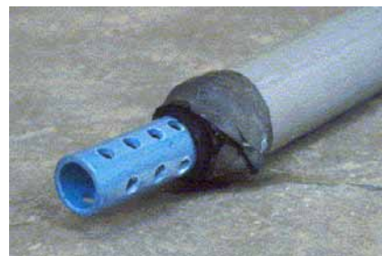
DTU valve fitted and sealed on to riser
