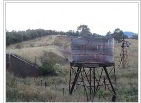
derelict windmill connected to water pump with water storage tank in the foreground
