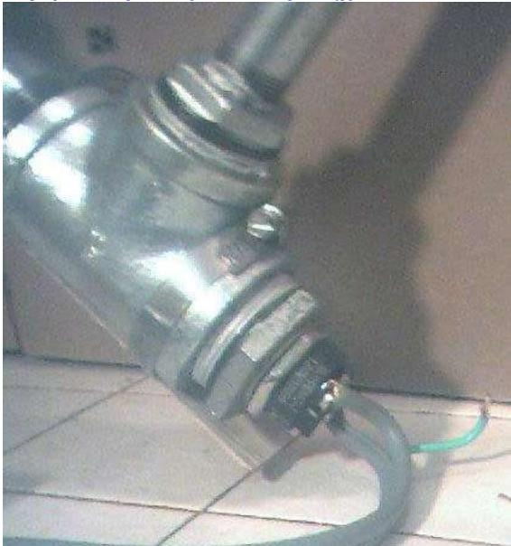
This is what the heater element fully installed looks like and with a wood strip held on with a hose clamp for bump protection. The ground wire is put under the hose clamp to ground the pipe assembly.
