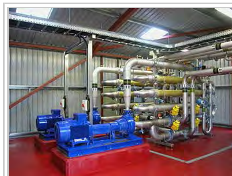
UF membrane side stream configuration
