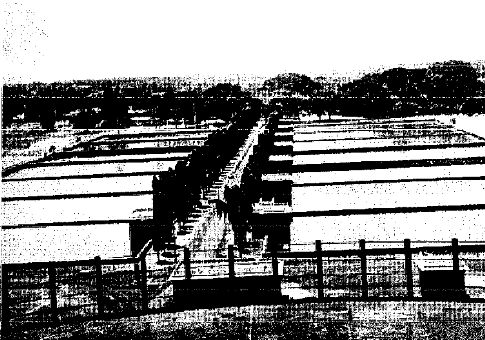
FIG. 2. SLOW SAND FILTERS AT MADRAS WATERWORKS, INDIA
