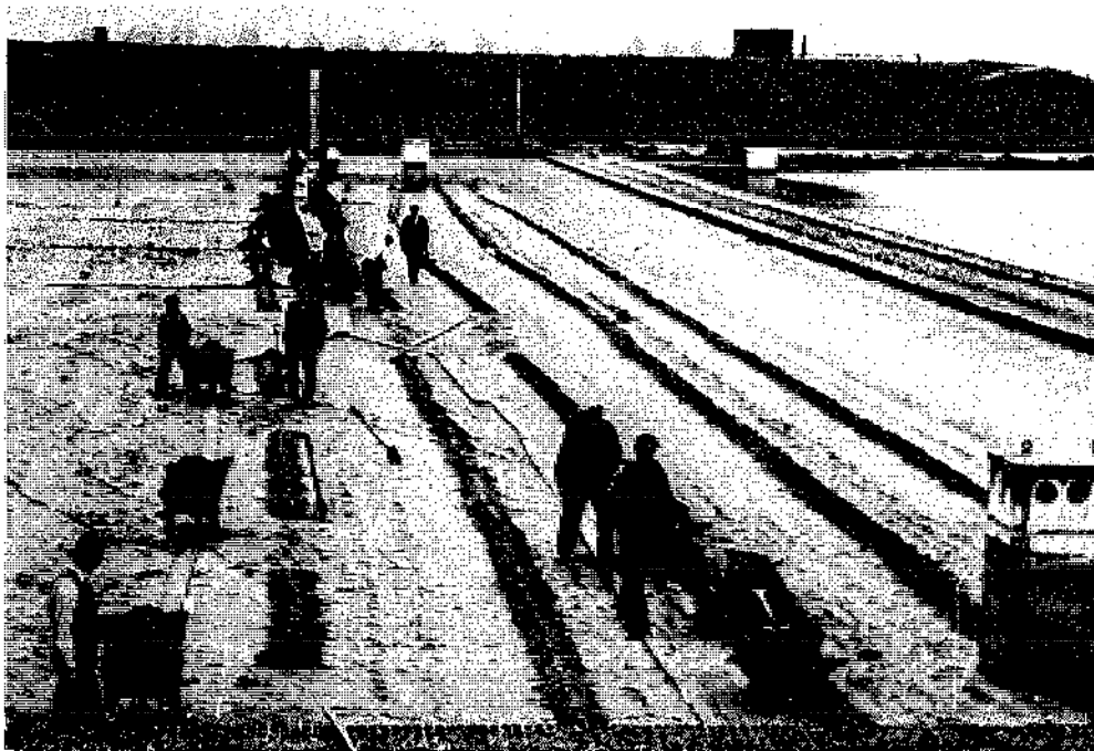
Municipal waterworks, Amsterdam
