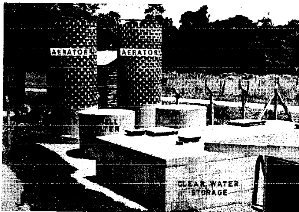
Note the shell filters for pH correction after filtration.
