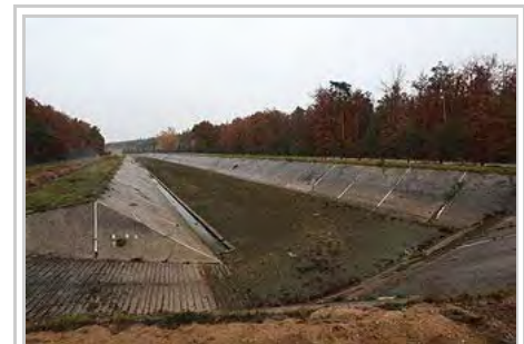
Slow "artificial" filtration (a variation of bank filtration) to the ground, Water purification plant Káraný, Czech Republic
