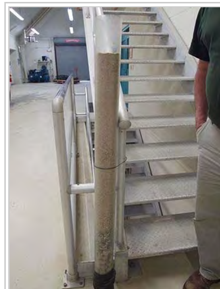
A profile of layers of gravel, sand and fine sand used in a slow sand filter plant.
