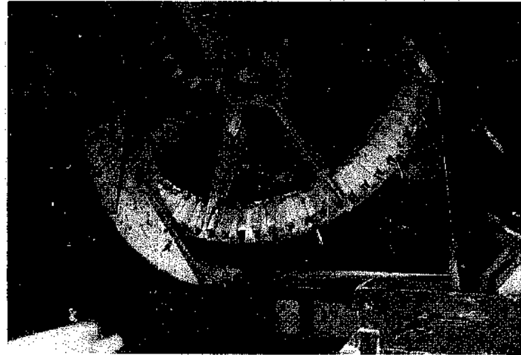
(b) Friston Post Mill, Suffolk (1938). Lever struck by tail wheel
