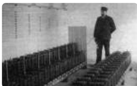
The battery store room of a wind power plant at the beginning of the 1900's • (H.C.Hansen: Poul la Cour)
