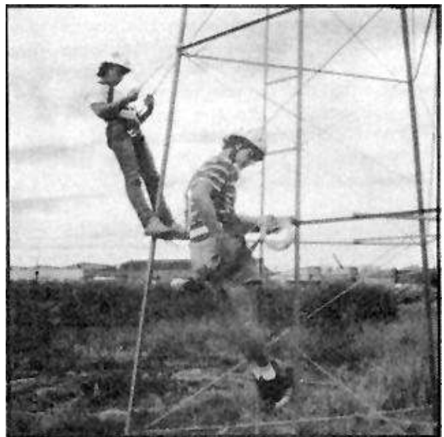
Hanging safely from the tower thanks to the safety harnesses
