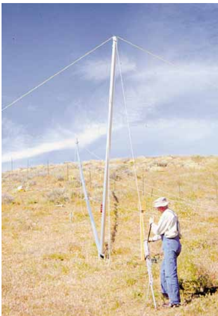
Below: The tower almost down. The forward lever on the griphoist is used to pay out cable.
