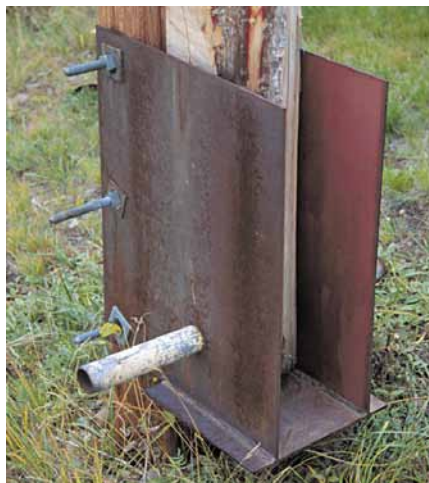
Above: Base detail showing 1/4 inch plate steel bracket, the shaved spar sides, and 1 inch pipe hinge.
