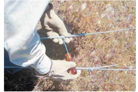
Above: Tightening wire rope clips. Remember, "Never saddle a dead horse."
