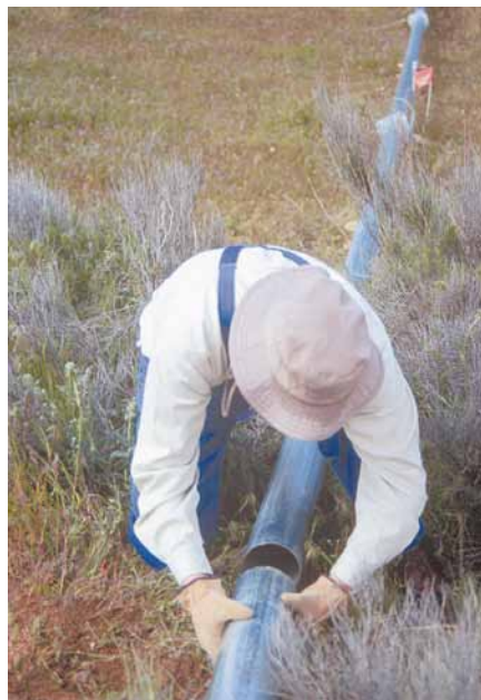
Above: NRG tower sections slip fit together and seat firmly when the tower is raised.
