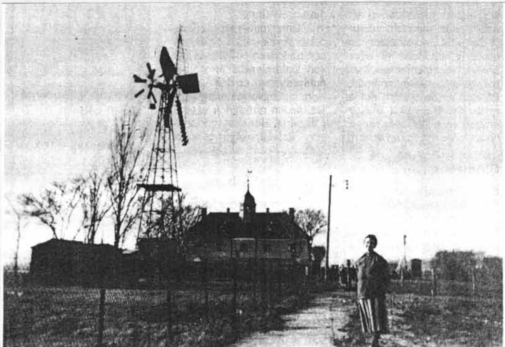
Wind-turbine of Type 1 - 1.5 built 1904. 10 kW DC Generator Tower height 17 m. Blade diameter 16 m. Sited in Copenhagen Harbour, in operation until 1957. This was a combined wind-turbine - petroleum spark ignition motor generator.
