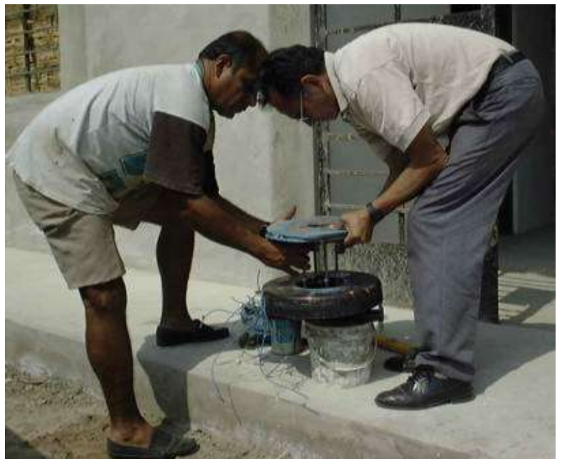
On site assembly in Peru
