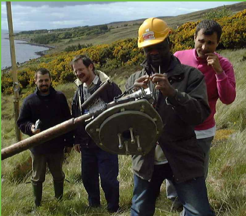
Pic 30: The last touch, tightening the blade assembly onto the alternator before raising the previously tested pole configuration, carefully of course.
