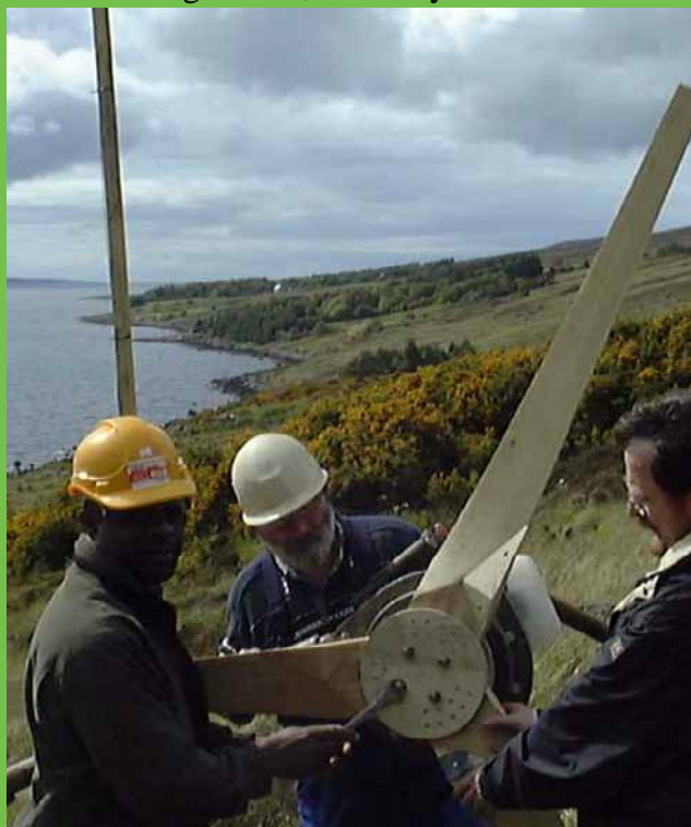
Pic 30: The last touch, tightening the blade assembly onto the alternator before raising the previously tested pole configuration, carefully of course.
