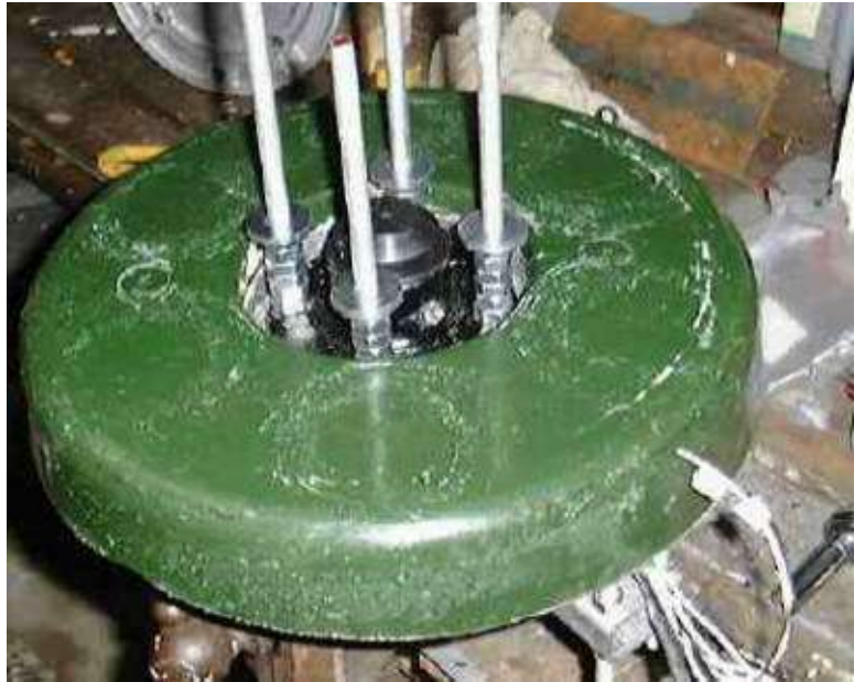
Fitting the stator
