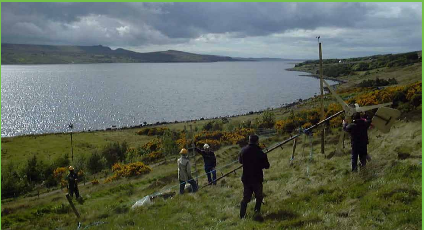
Pic 33: We were all looking - somewhat in awe - at the wind turbine we started building from scratch just 5 days ago actually generating electricity. What a rewarding moment!(We had an anemometer to check the windspeed. It was mostly around 3-5 m/s (7-11 mph) Output was around 20-100 watts. Hugh)
