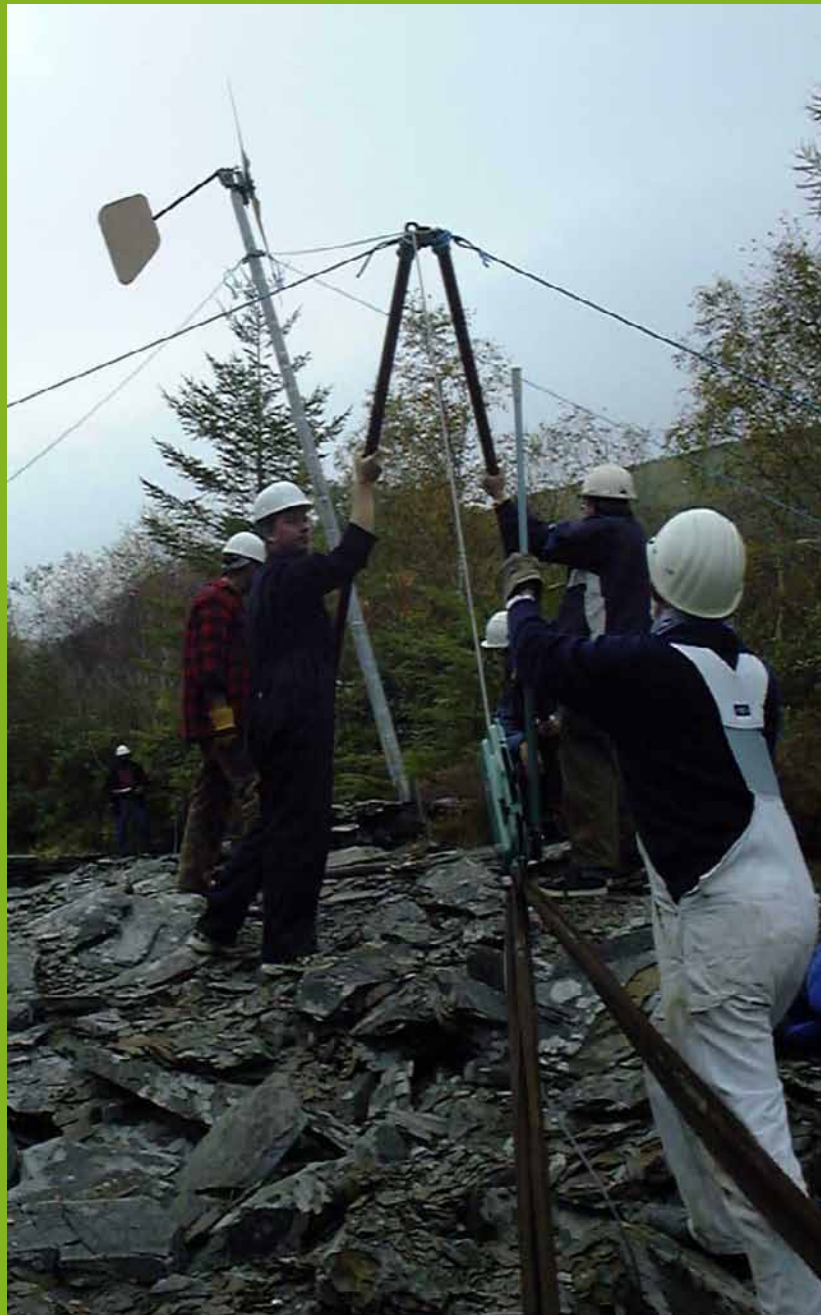
Erection on site at CAT.
