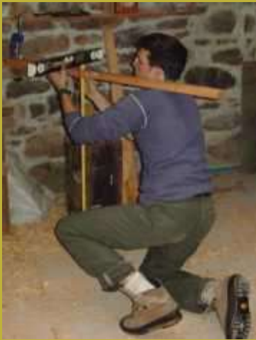
Checking the blade angles using a spirit level and ruler.
