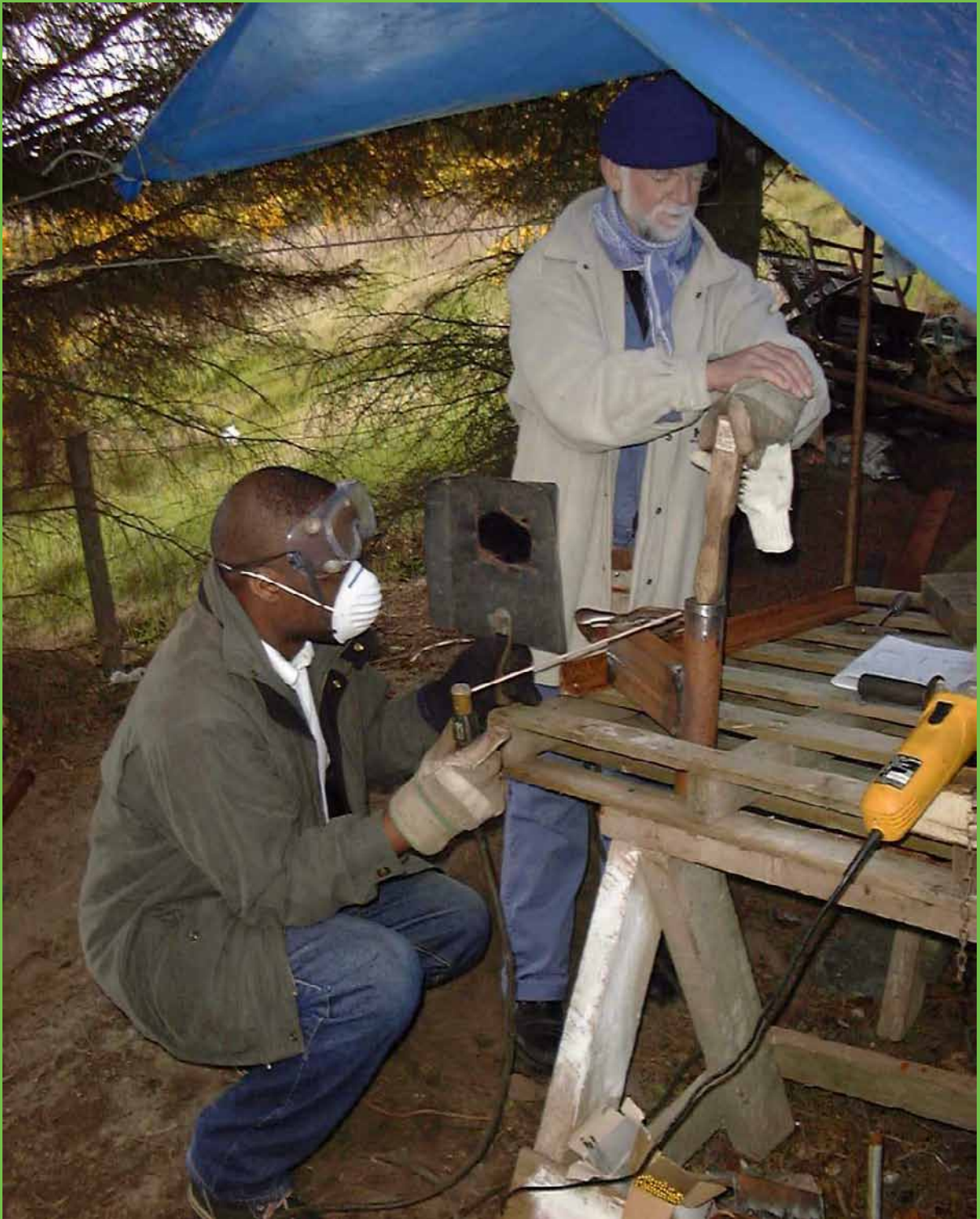
Pic 12: Demian also proved to be a talented welder. These little gas powered generators can become real life savers when everything else fails. A litre or less of petrol and you can do all the welding, cutting, lighting, you name it!
