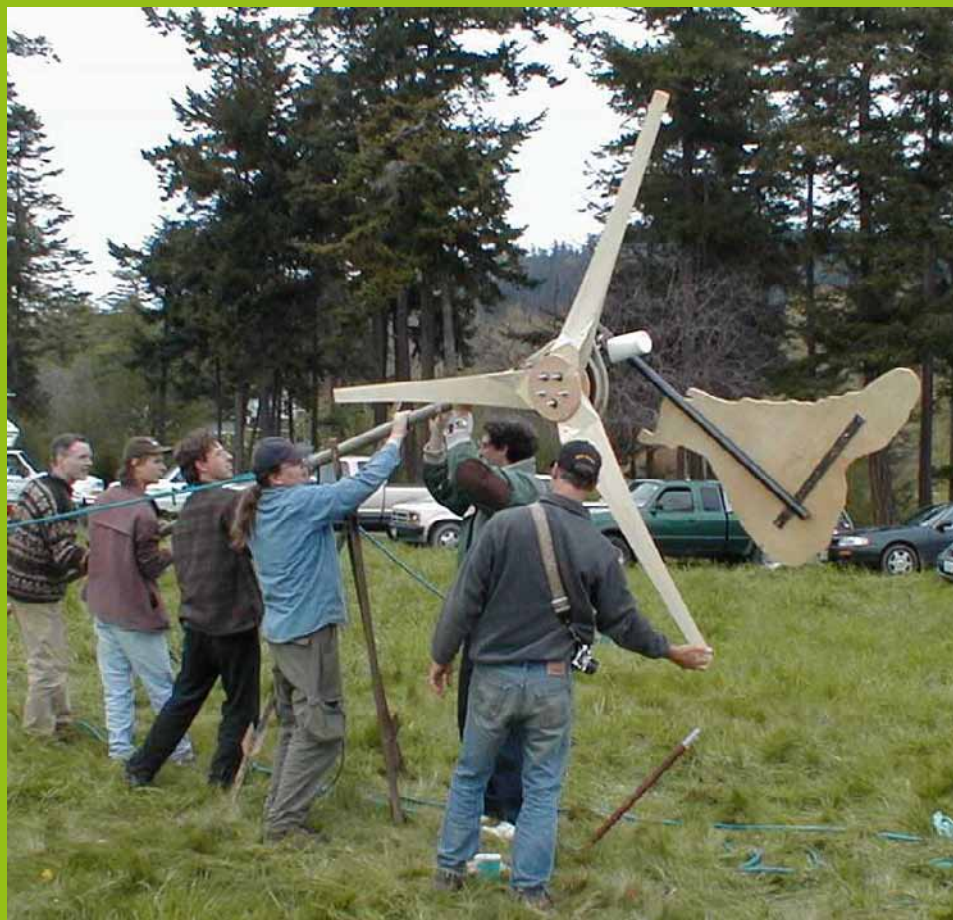
Putting the larger machine onto the tower for erection. The tail is a map of the island.
