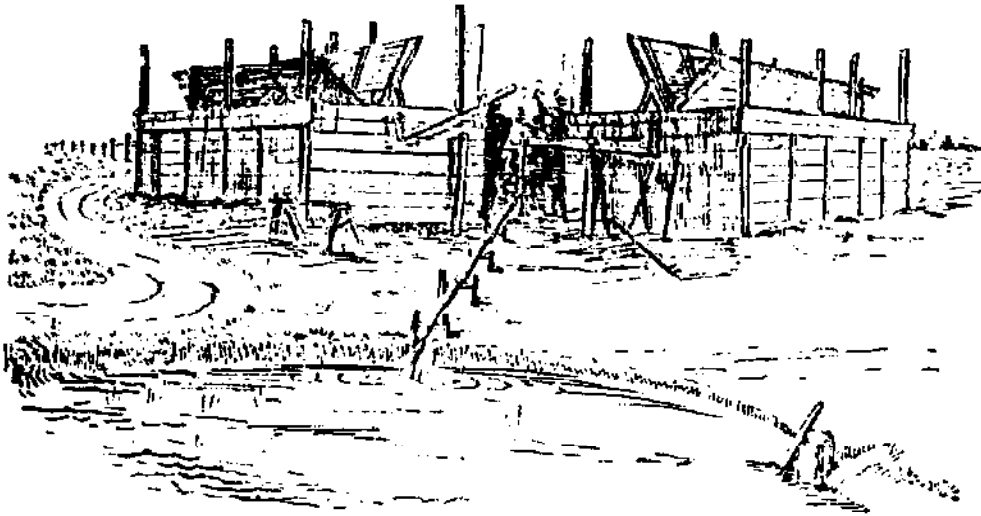
FIG. 23. Sometimes Jumbo windmills are built in pairs, one standing north and south, the other east and west, so as to insure service whatever the direction of the wind.
