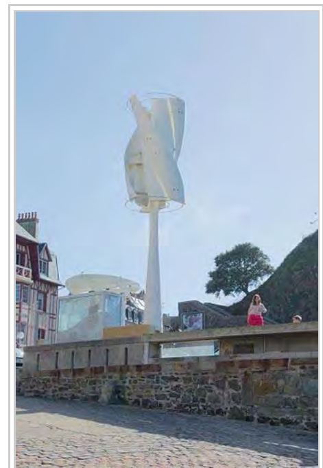
Twisted savonius wind turbine in Granville, France
