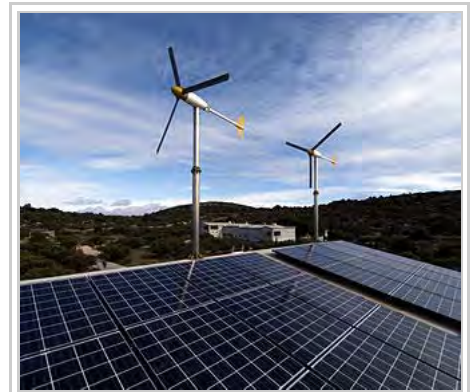
Hybrid system, 2400W windturbines, 4000W solar modules, island Žirje, Croatia [19]
