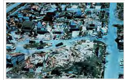
Damage from Hurricane Andrew
