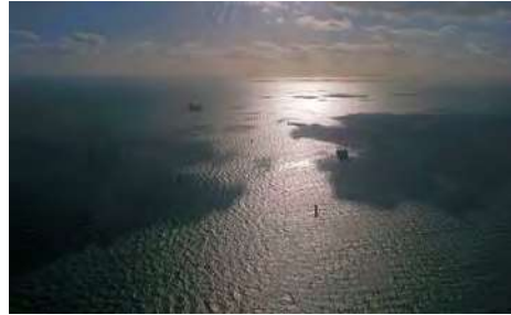
The London Array under construction in 2009
