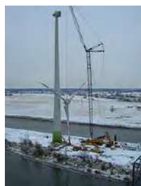
Erection of an Enercon E70-4 in Germany.
