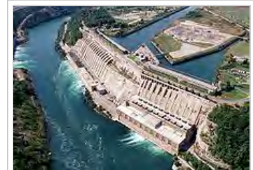
The Sir Adam Beck Generating Complex at Niagara Falls, Canada, includes a large pumped-storage hydroelectricity reservoir. During hours of low electrical demand excess electrical grid power is used to pump water up into the reservoir, which then provides an extra 174 MW of electric power during periods of peak demand.
