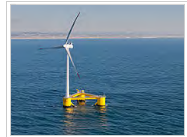
The world's second full-scale floating wind turbine (and first to be installed without the use of heavy-lift vessels), WindFloat, operating at rated capacity (2 MW) approximately 5 km offshore of Póvoa de Varzim, Portugal
