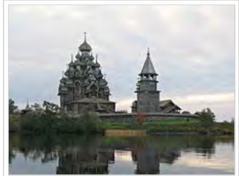
The churches of Kizhi, Russia are among a handful of World Heritage Sites built entirely of wood, without metal joints. See Kizhi Pogost for more details.
