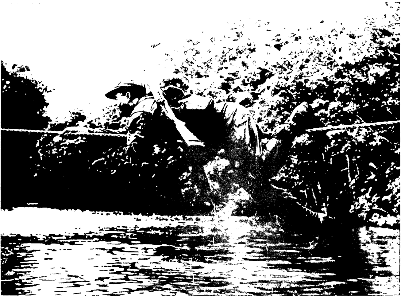
Figure 99. Single strand rope bridge. Soldier is shown crossing a narrow, deep jungle river using the "British Crawl" method. It is important that the soldier push with the foot on the rope as well as pull with his arms to conserve strength.
