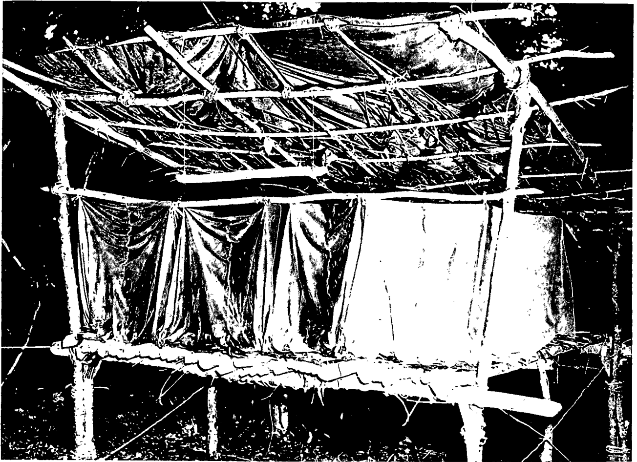
Figure 34. Four-man shelter using two ponchos as a hasty roofing expedient.
