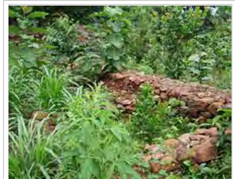
Walls built to avoid water run-off
