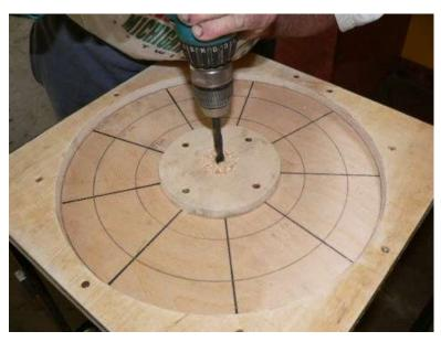
Drill a 7/16" diameter hole all the way through the center of the mold. tapping this hole for the threaded rod - since it's wood you could use a smaller drill bit, the tap will cut wood easily.
