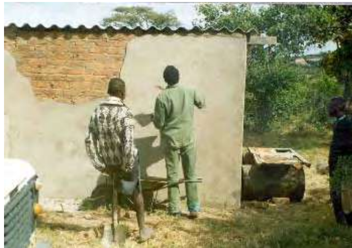
Fig 29 Plastering and sealing a storeroom to ensure it is rodent proof
