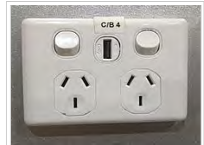
Australian and New Zealand power socket with USB charger socket
