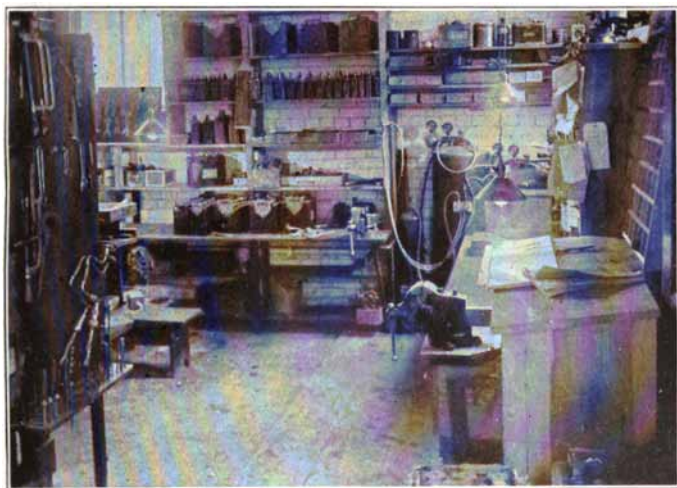
Fig. 53. Corner of Workshop, Showing Burning Outfit, Burning Bench and Vises
