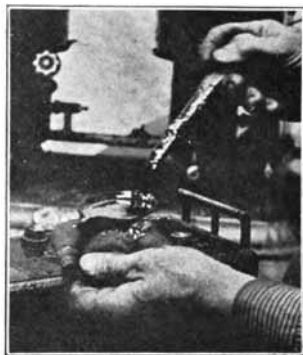
Fig. 150. Wiping Bottom of Spoon Filled with Sealing Compound
