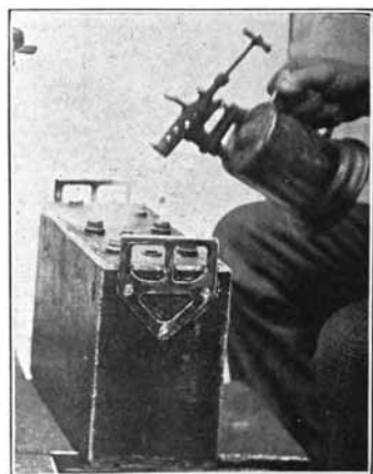
Fig. 103. Heating Compound with Torch
