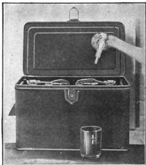
Fig. 26. Release the Pressure on the Bulb and Hold Syringe in a Horizontal Position to Prevent Water from Dripping on Battery. Return Excess Water to Glass
