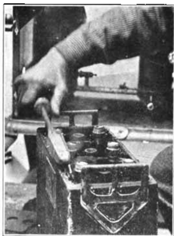
Fig. 145. Using Very Hot Sealing Iron Around Case
