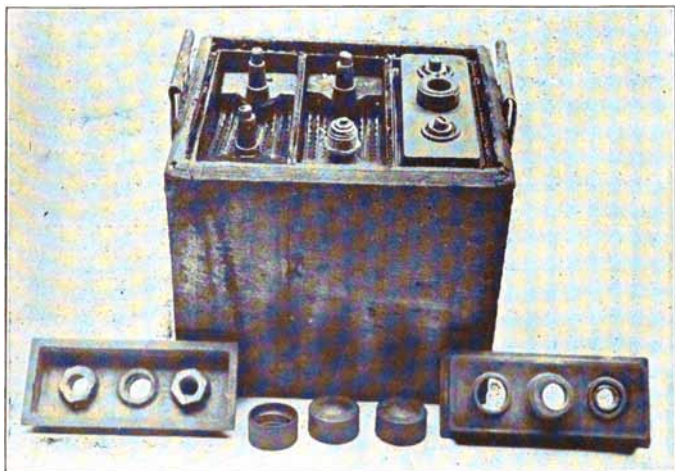
Fig. 181. Prest-O-Lite Battery, Showing Parts and Construction
