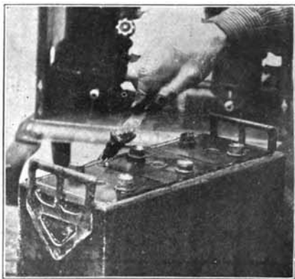
Fig. 152. Final Operation of Cleaning Off Compound with Putty Knife to Make It Flush with Case and Top Covers
