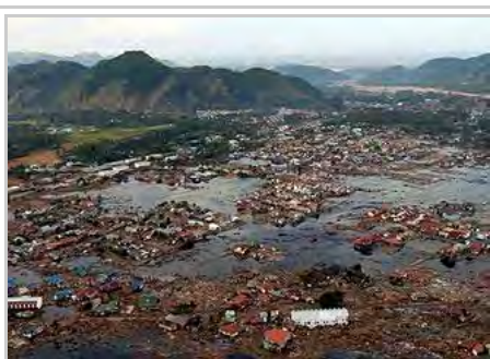
A town near the coast of Sumatra lies in ruin after the 2004 Indian Ocean earthquake and tsunami.
