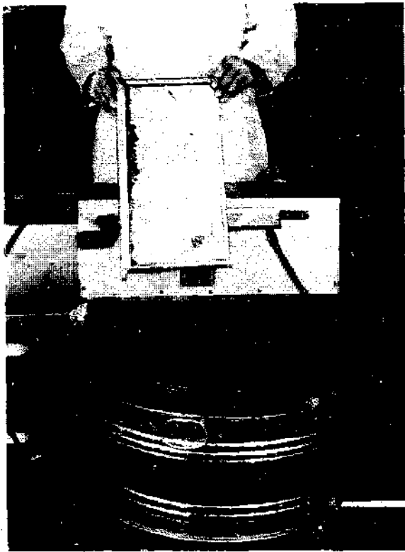
One-blade power uncapping machine. Part of the honey drains into the tub and is pumped directly into the storage tank. Note the pipe at the bottom leading to the honey pump.
