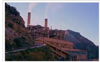
Castle Gate Power Plant near Helper, Utah, USA
