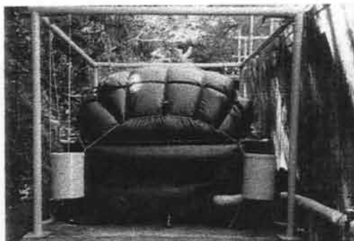
Pilas Coffee Mill: biogas bag (10 m 3 )
