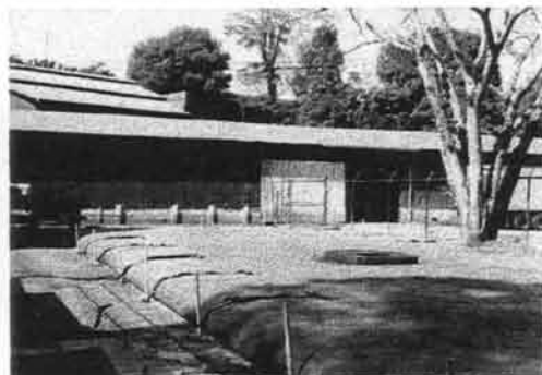
Pilas Coffee Mill: waste water storage (400 m 3 )
