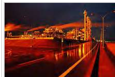
An oil refinery in Mina-Al-Ahmadi, Kuwait
