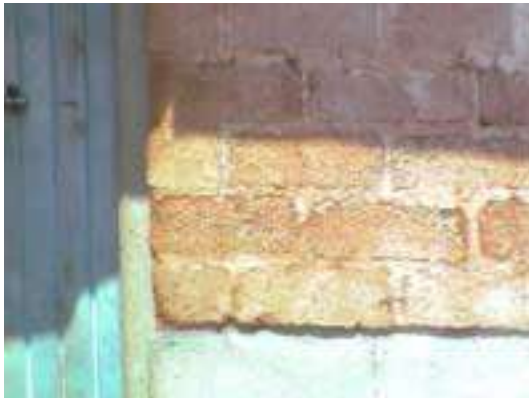
Balram block walling (self build)
