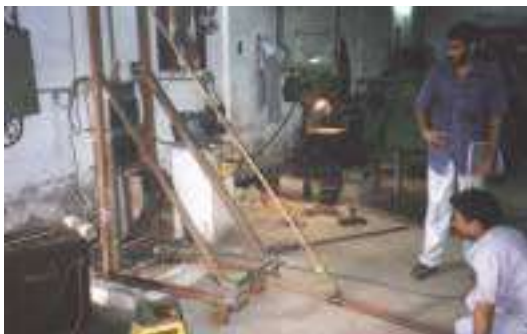
Impactor lifting mechanism added
