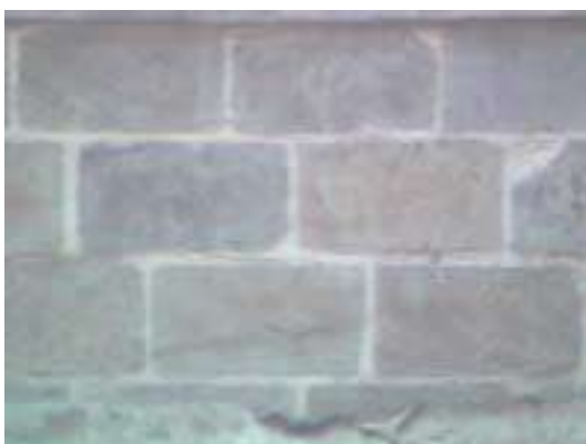
Stone cladding over bricks
