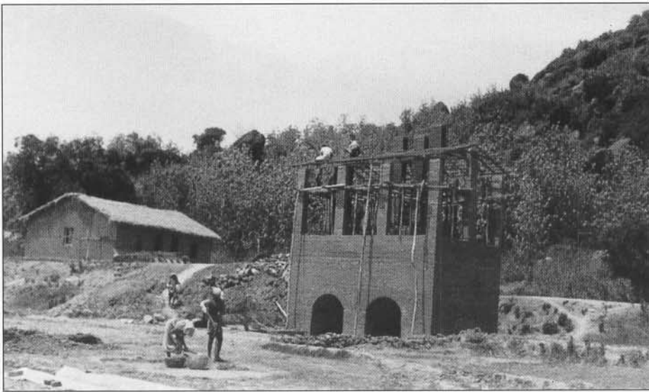
Fig. 4: Kiln construction nearing completion May 1997
