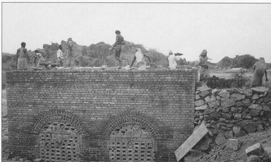
Fig. 3: Kiln construction at the level of the loading platform
