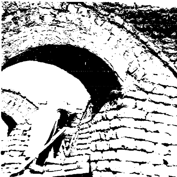
FIGURE 15. The mason is just beginning the construction of the vaulting in the corner of a room. The guide stick to insure that each course is circular is in use. In the foreground may be seen the vaulting, the pendentives, completed. A hemispherical dome will complete the roof structure.
