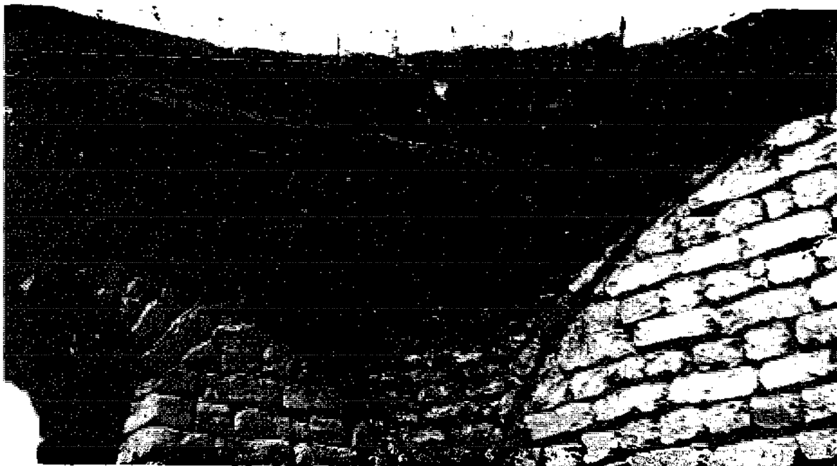
FIGURE 16. Low dome construction in mud brick without centering. The minimum height of the house is established by the supporting structure above the opening. The triangular vaulting in each corner carries the dome.
