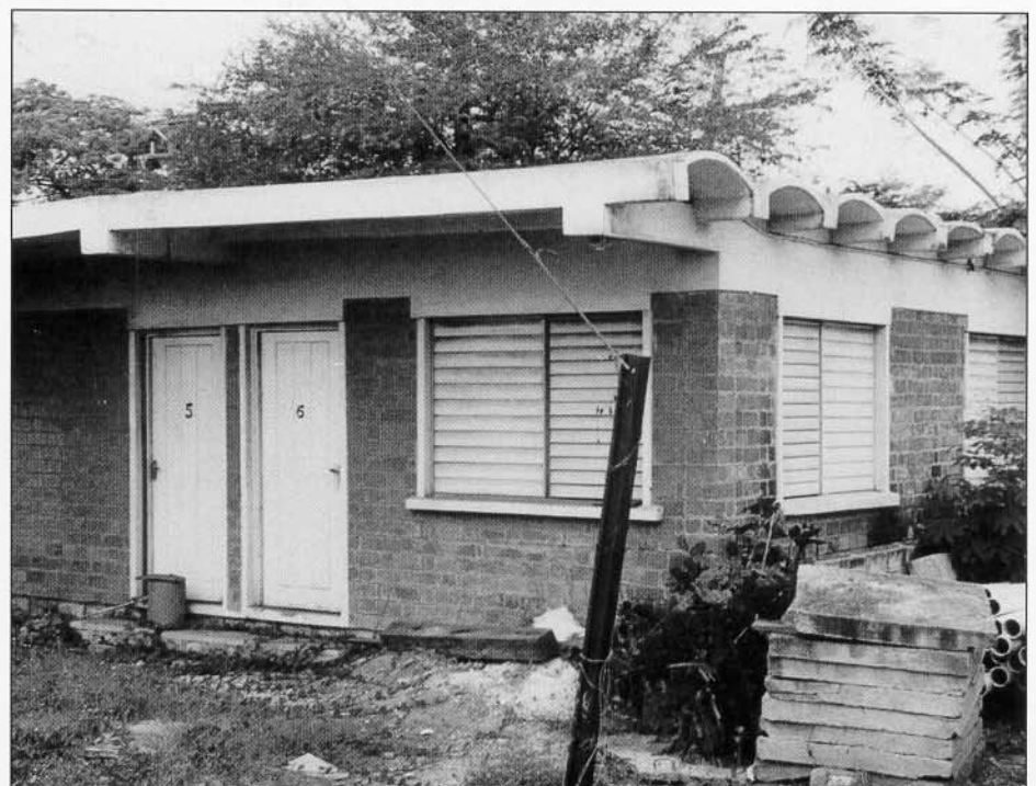
Fig. 4: The BRI red mud demonstration building (1998)
