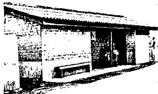
Clinic built at Kabiro, Kenya with 'BrePak' Soil Blocks
