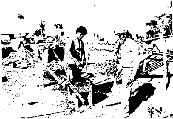
Placing the dividers before filling the moulds.
