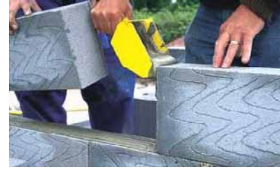
C – Thin mortar joints
