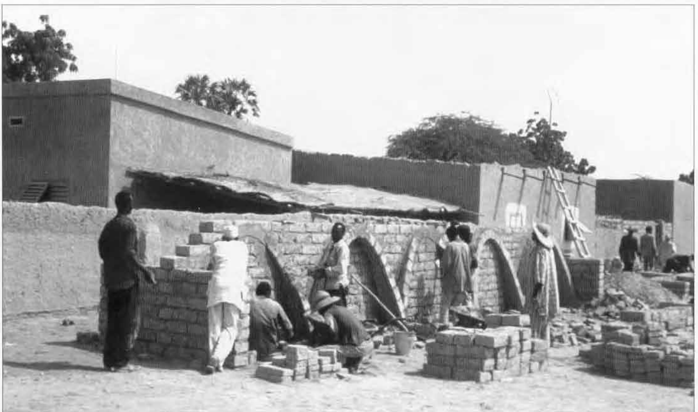
Figure 1 Trainee masons practice starting off vaults on training structures (phase 2)
