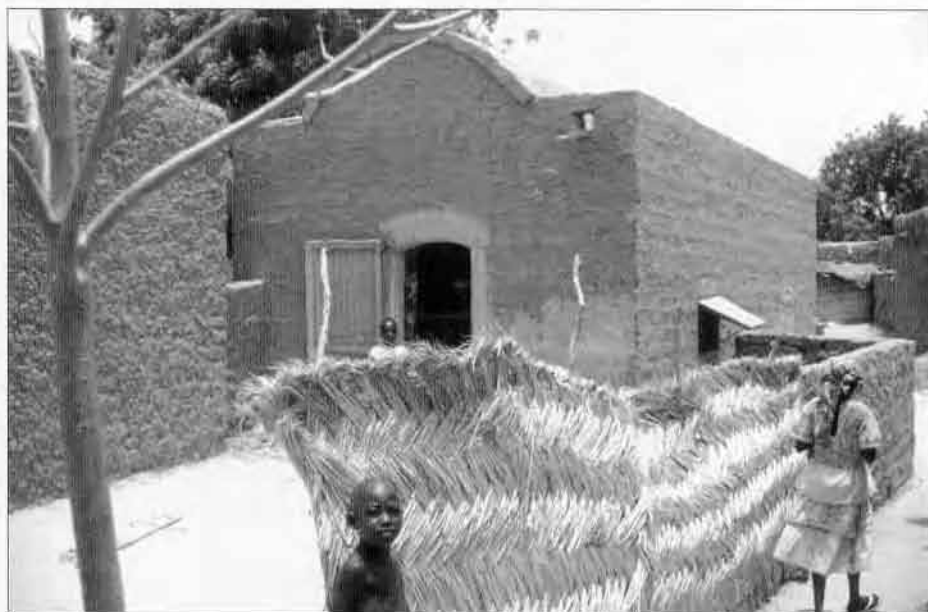
Figure 4 "Spontaneous" construction – a vaulted house built by a trained mason with no external help
