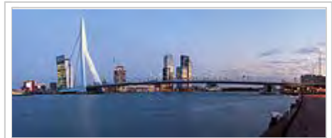
Erasmus Bridge, Erasmusbrug, in Rotterdam, Netherlands
