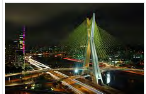
Octavio Frias de Oliveira bridge, in São Paulo, Brazil. It is the only bridge in the world that has two curved tracks supported by a single concrete mast.
