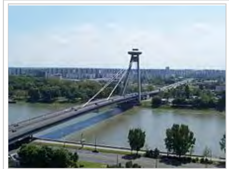
Most SNP (Bridge of the Slovak National Uprising) - the world's longest cable-stayed bridge to have one pylon and one cable-stayed plane (Bratislava, Slovakia, 1967-1972).
