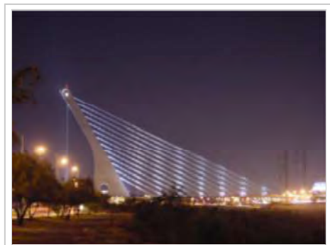
Puente de la Unidad, joining San Pedro Garza García and Monterrey, a Cantilever spar cable-stayed bridge
