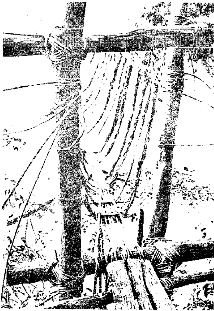
Fig. 3 Woven palm leaves suspended from the main structure of a bridge at Taka, Papua New Guinea, Papua New Guinea.
