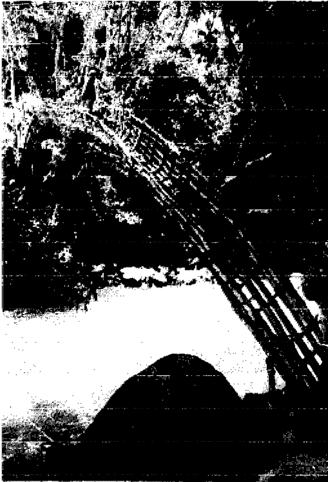
Fig. 77 Sau River Bridge. Note cane suspended cables supporting the middle of the bridge.
