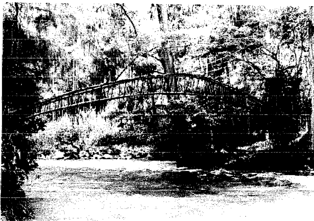
Fig. 59 Kubib Bridge over Mendi River, seen from the east bank looking south.
