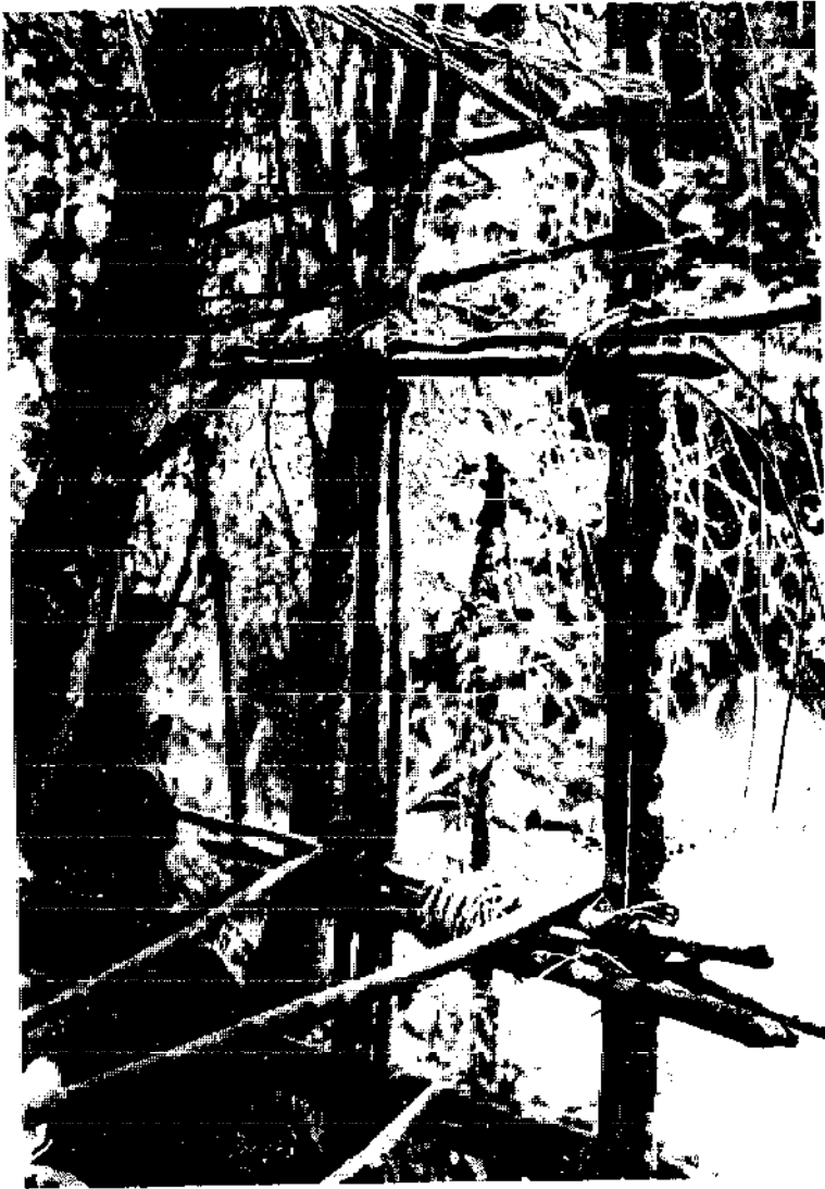
Fig. 86 Nepirik Bridge, east anchorage, using trees for additional support.
