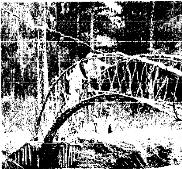
Fig. 95 Close-up of the walkway, showing vine lashing and suspenders, Saimanda Bridge.
