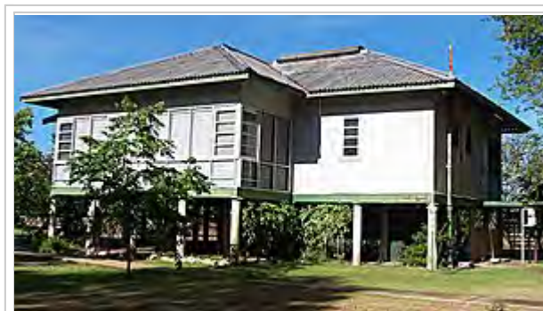
A pre-WW2 house in Darwin. The roof is sheeted with corrugated fibro sheets and the walls with flat fibro sheeting, with fibro battens covering the joints.
