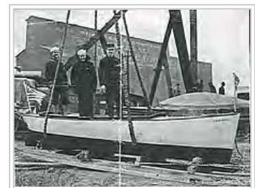
Concrete boat constructed by Walter Dowsey hauled out in Chicago
