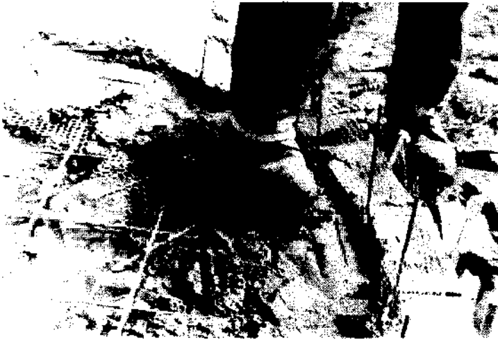
5.2 Tread mortar into corner.
