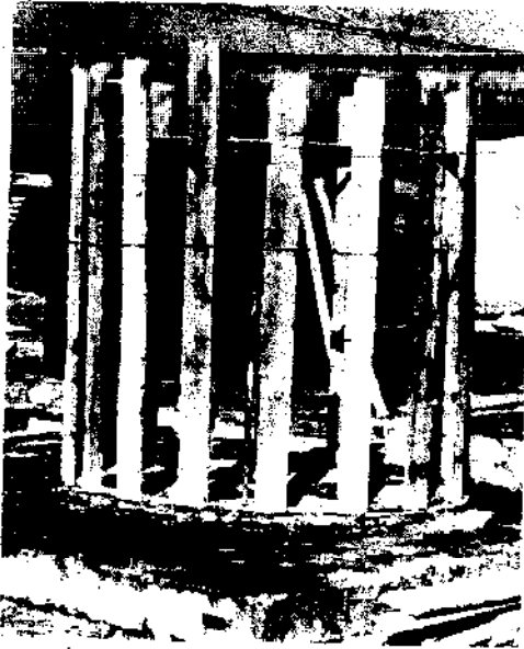
3.1 The inside former, which provides the tank shape, is usually a series of vertical planks supported by a steel frame. These will be sheathed in sheet steel before applying the plaster.
