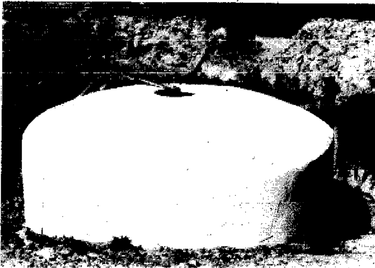
9.8 Finished tank with inlet.
