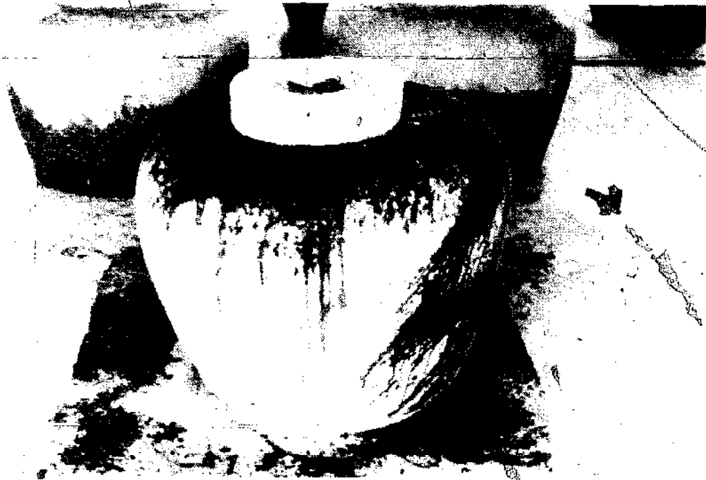
2.7 Place a circular ring on the top of the sack to make a mould for the opening of the jar. This can be made of wood or precast mortar.
