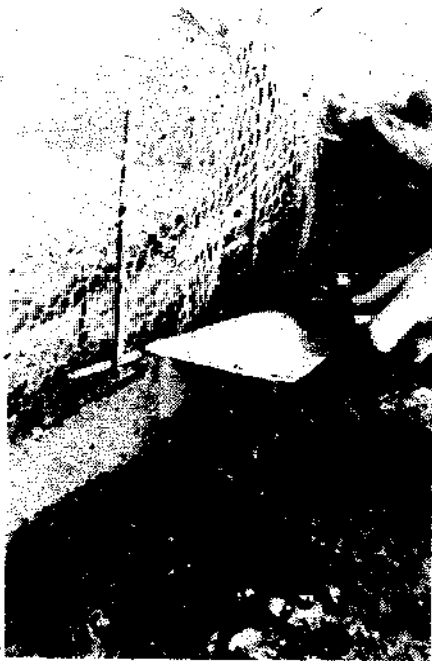
5.4 Bend up reinforcement
