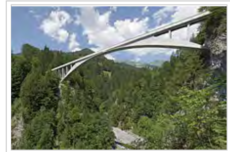
Salginatobel Bridge, Switzerland.
