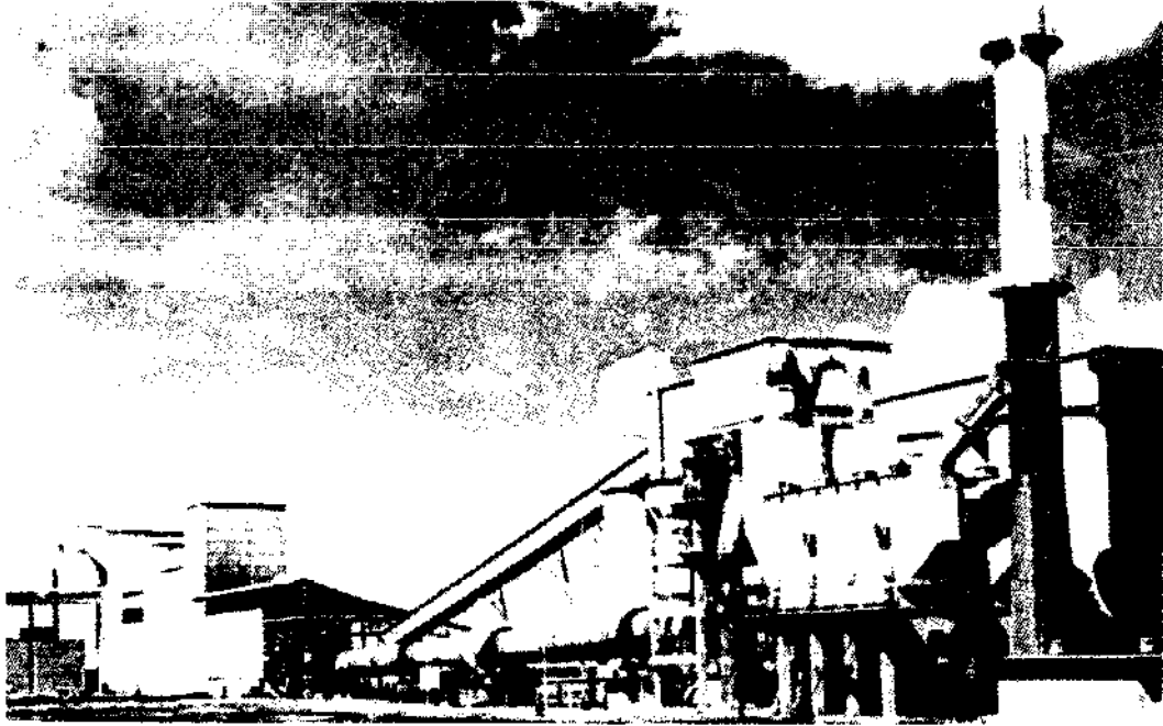
Fig 1. Cement plant at Ndola, Zambia Capacity 600 tonnes/day (Photo by permission of the Chilanga Cement Co)
