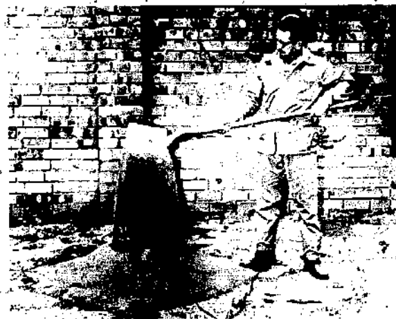
Fig. 26 Adding cement to the soil.
