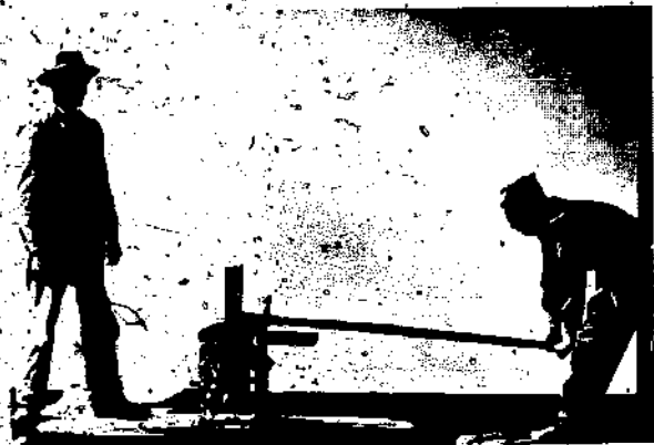
Fig. 37 (c) - Maximum compaction of the block.
