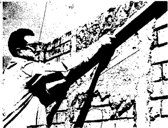
Fig. 91 Using the scraper in plastering a wall.
