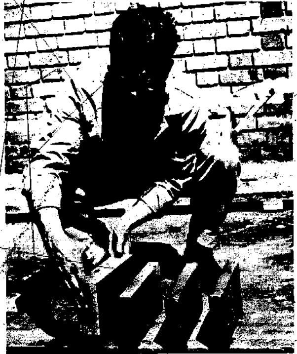
Fig. 93 Removing the tile
