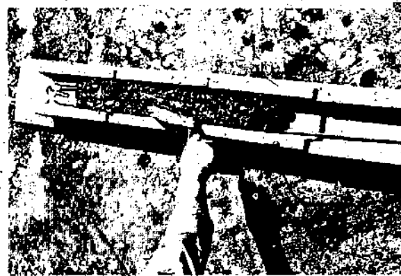
Fig. 68 Lintel prefabricated in U-blocks.
