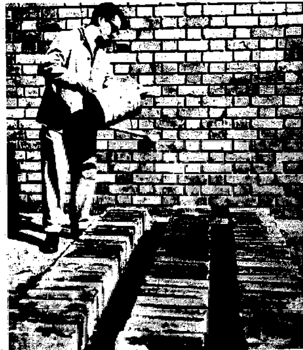
Fig. 40 Watering the blocks.
