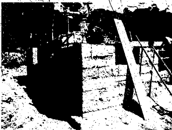
Fig. 70 Three types of shuttering for monolithic walling.
