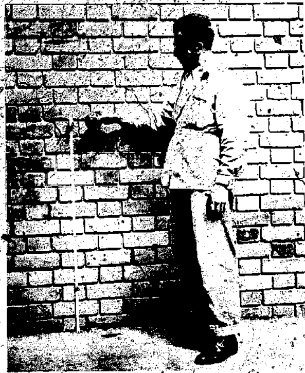
Fig. 29 (a) The right amount of water: dropping test.
