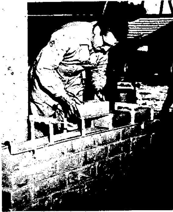
Fig. 58 Laying soil-cement blocks with a "block fitter".
