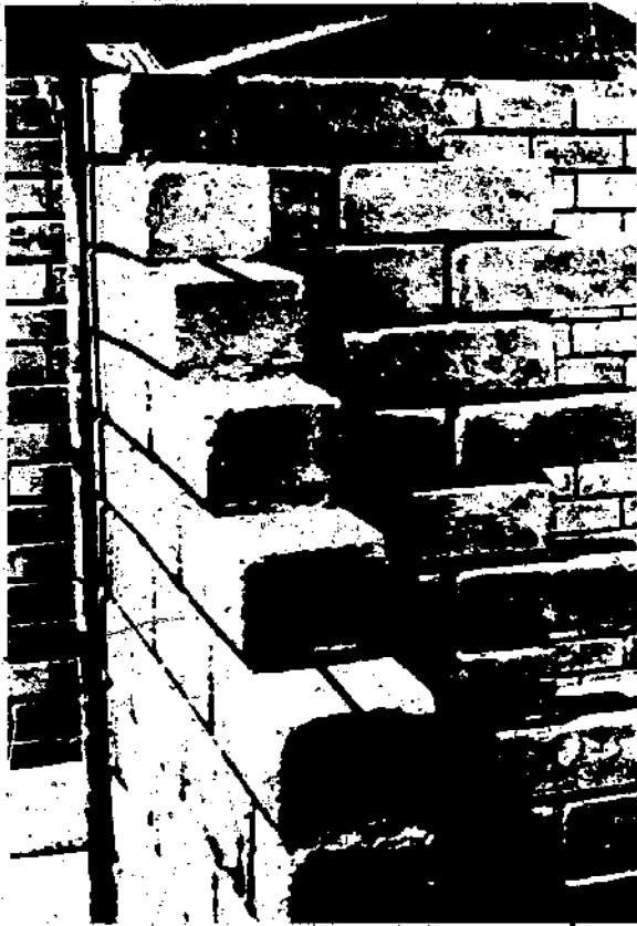
Fig. 66 Extra metal reinforcements for walls of soil-cement blocks are highly desirable in active seismic regions.
