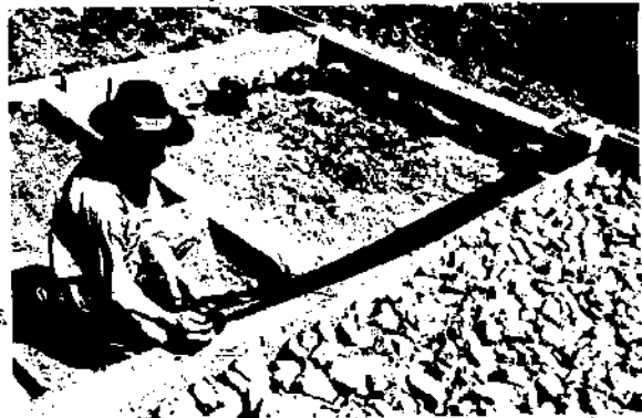
Fig. 55 Damp course of bituminous felt.
