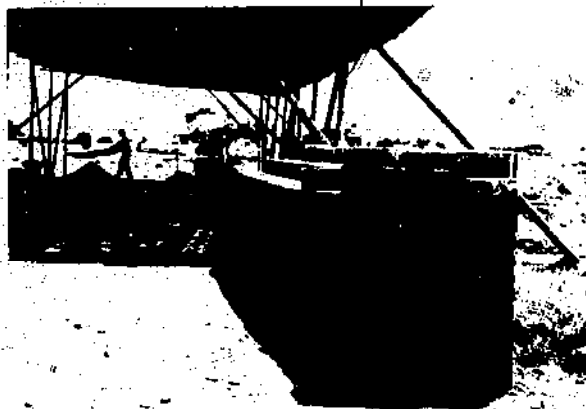
Figs. 39 and 39 (a) Drying and curing the blocks. Newly-made blocks are kept under cover. Stacked blocks.
