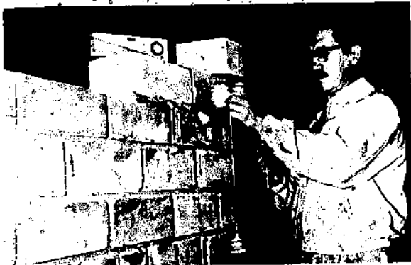
Fig. 56 Building a wall of soil-cement blocks.
