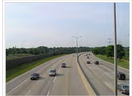
A highway paved with concrete.
