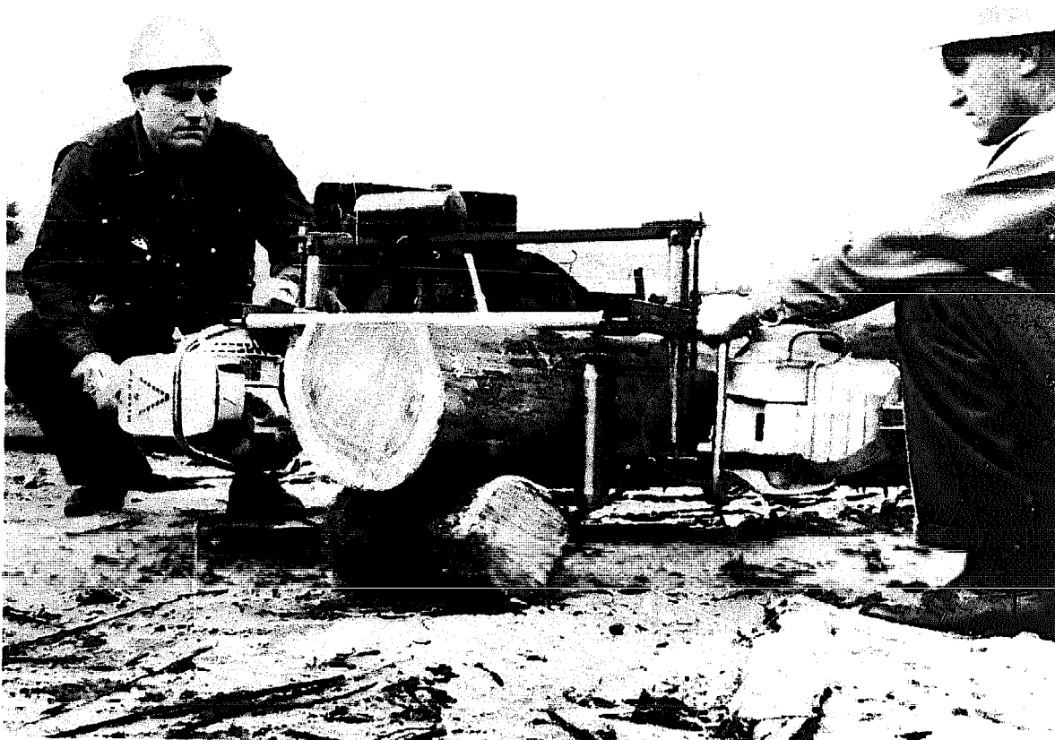
Granberg Alaskan Mill in operation
