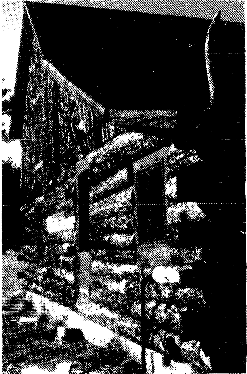
Barnacle Papp's slab and log cabin in Reed Gulch, Colorado
