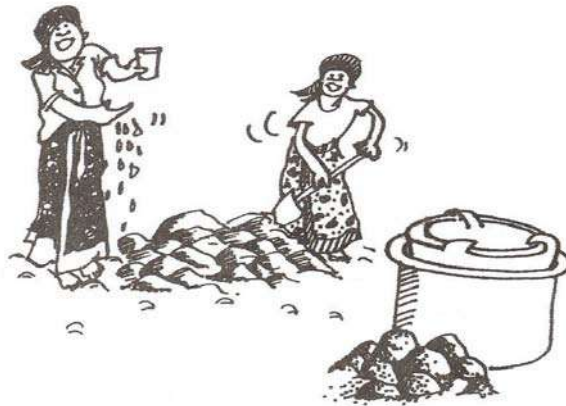
Fig. 7.2 Mixing murrum with water
